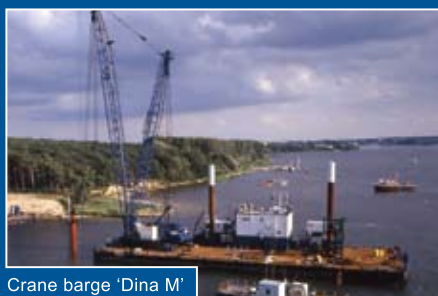
Crane barge 'Dina M'
